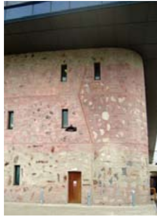
Tremough Elvan set in concrete
