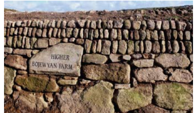
Cornish hedging using granite
