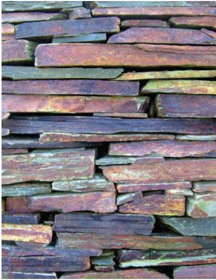
Dry walling - Delabole
